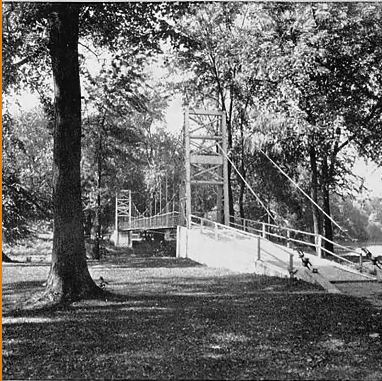
MEMORIAL BRIDGE, TIPPECANOE RIVER, WINAMAC, INDIANA
